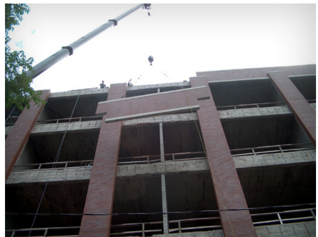
Installation of precast single wythe wall panels. Source: CPCI
