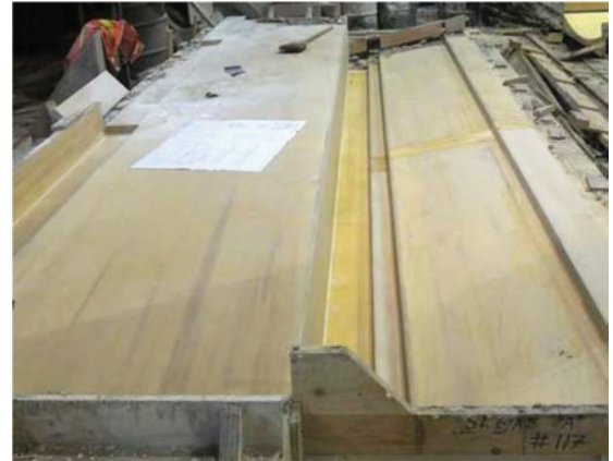
Combination of Envelope and Conventional Form (Only One Side is Removed for Stripping). Source: CPCI
