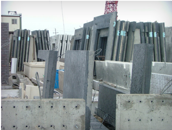
Storage of precast panels in yard. Source: M. E. Hachborn Engineering
