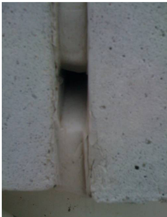
Vent and weep opening in sealant. Source: M. E. Hachborn Engineering
