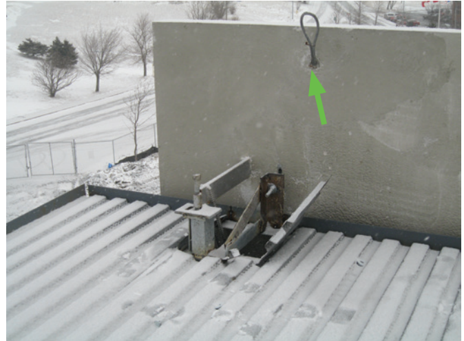
Lifting Loop (arrow) Source: M. E. Hachborn Engineering
