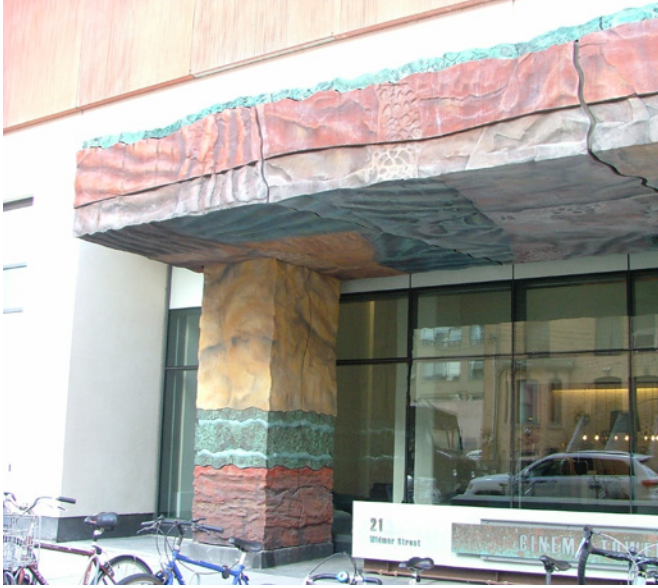
Surface applied stain can be used for interesting architectural effect. Source: M. E. Hachborn Engineering
