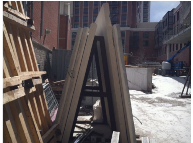
Storage of precast panels on site. Source: CPCI
