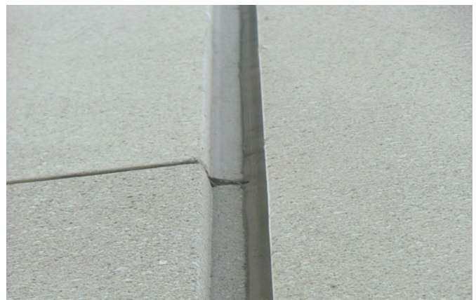
Recessed or Reveal Joint. Source: CPCI
