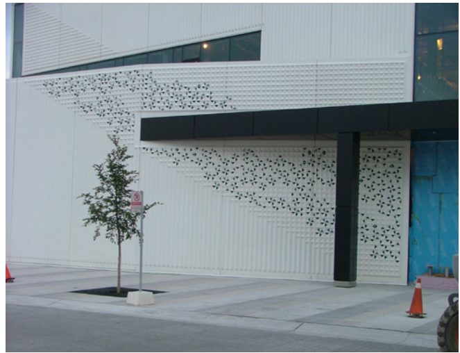
Form liners can be used to create interesting visual effects. Source: M. E. Hachborn Engineering
