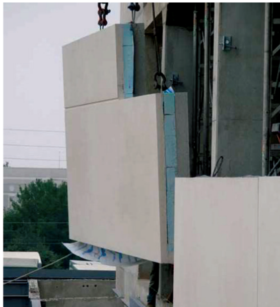
Double wythe precast concrete insulated wall panel being installed. Source: CPCI
