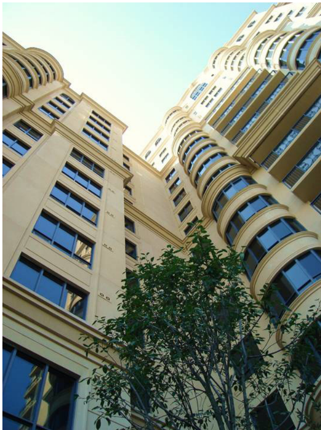
Multi-unit residential precast cladding. Source: M. E. Hachborn Engineering
