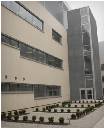
Alternating bands of Precast Panels and Windows. Source: CPCI
