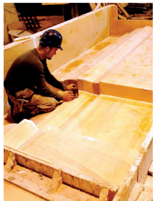
Manufacturing with a conventional form. Source: CPCI
