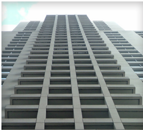
Precast horizontal panels with column covers. Source: M. E. Hachborn Engineering
