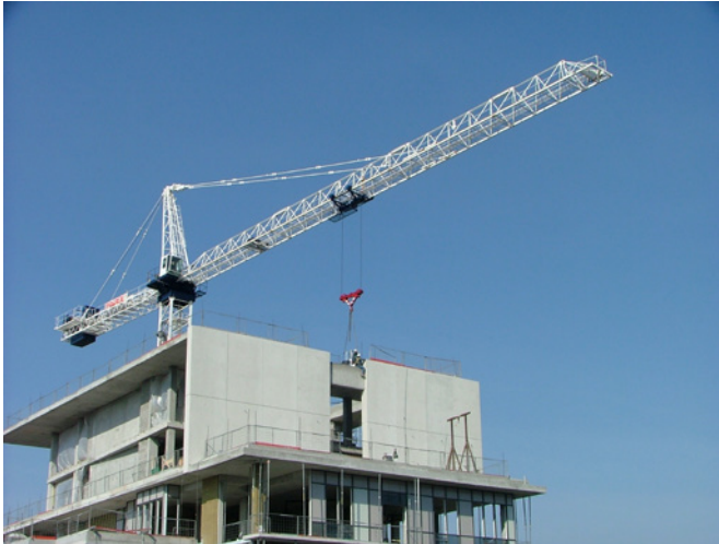
Erection of a precast panel using a tower crane. Source: CPCI
