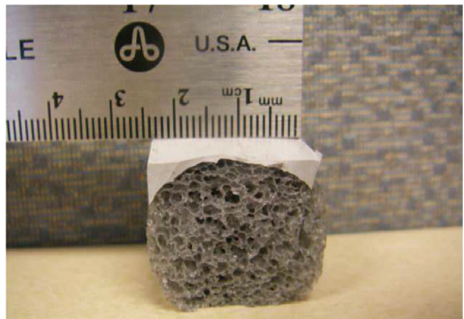
Sample testing of installed sealant to confirm proper dimensions. Bead is far too thin at the center, and bond edges are too narrow in this instance. Source: Morrison Hershfield
