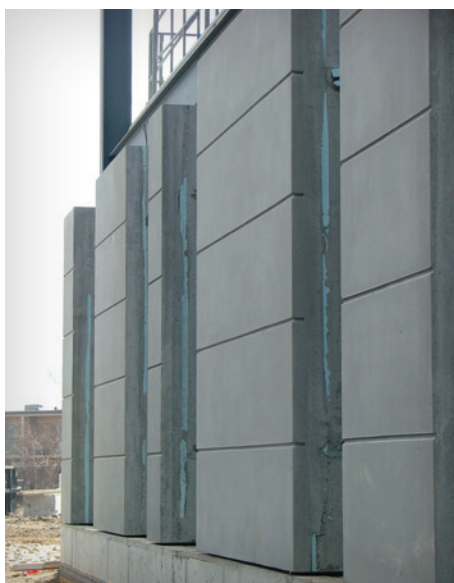
Double wythe precast concrete insulated wall panel. Source: CPCI
