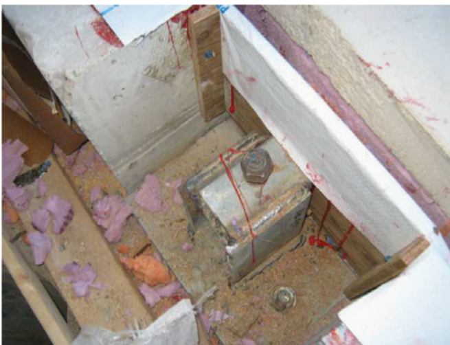
Precast panel connection prior to encapsulation to prevent thermal bridging. Source: Morrison Hershfield
