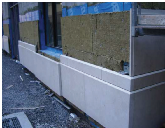
Handset precast panels installed in a drained wall system. This approach might be necessary for retrofit projects but is discouraged for new projects. Image copyright RDH Building Science Inc., used with permission
