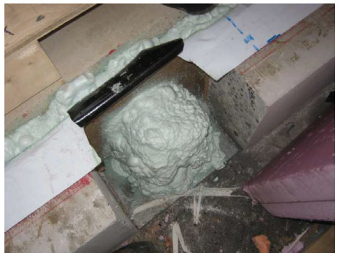
Precast panel anchor after spray foam encapsulation to prevent thermal bridging. Source: Morrison Hershfield
