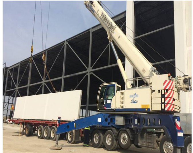
Lifting precast panel from transportation truck. Source: Numesh Inc.
