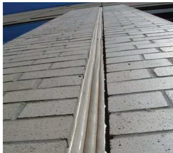
Expandable foam expansion joint material. Source: Emseal Corp.
