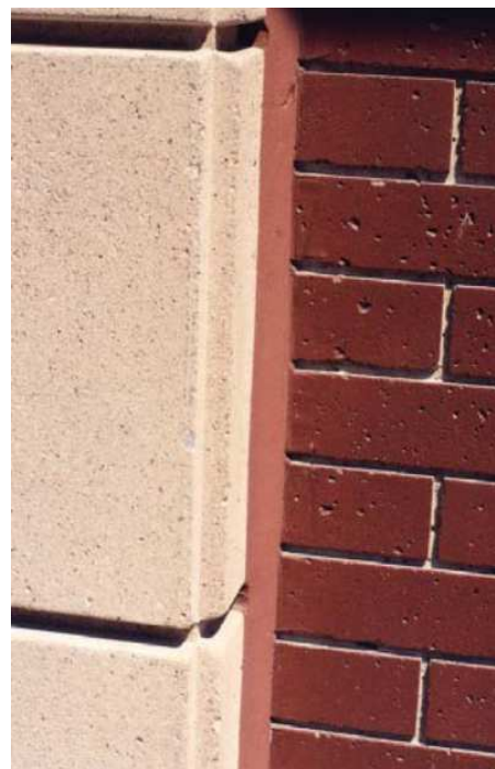
Good quality sealant joint between precast panels. Source: CPCI
