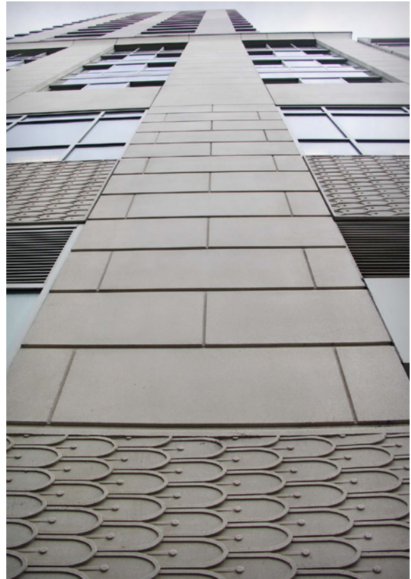
A variety of visually pleasing patterns and textures can be created with architectural precast wall panels. Source: CPCI
