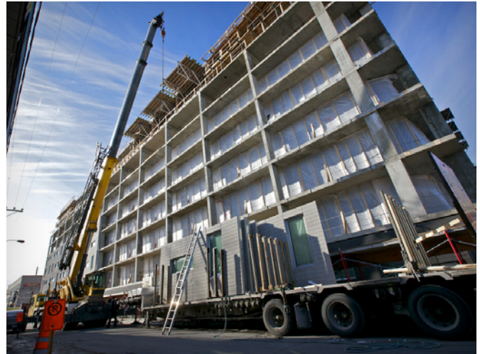
Erection of a precast panel using a mobile crane. Source: CPCI
