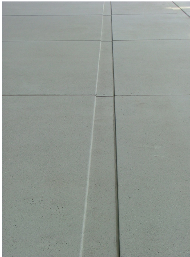
Precast wall alignment. Source: M. E. Hachborn Engineering
