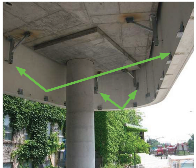
Lateral tie anchors. Source: Morrison Hershfield
