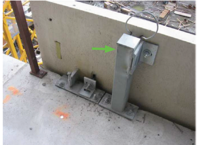
Eccentric lateral load connection. Source: Morrison Hershfield
