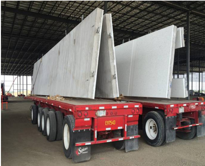
Transportation of precast panels. Source: Numesh Inc.
