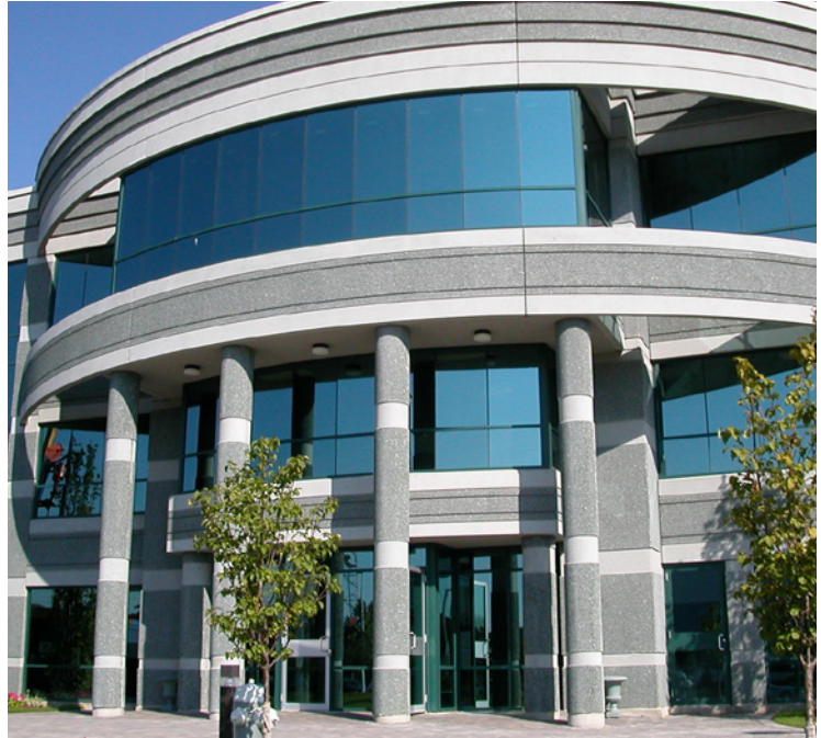
Precast panel where the aggregate has been exposed over a portion of the face by washing. Source: CPCI
