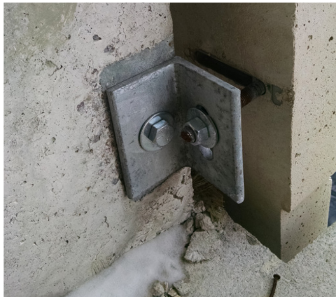
Lateral tie anchors. Source: Morrison Hershfield
