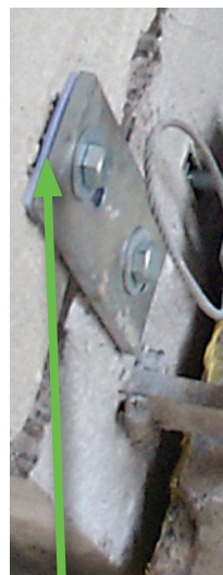
Shim placement for aligning panels. Source: M. E. Hachborn Engineering
