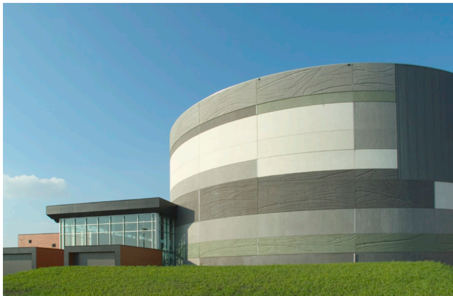
Solid wall panels with alternating patterns of smooth and ribbed textures. Source: CPCI
