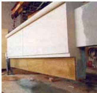
This detail view shows stone veneer on precast that was used as a window surround.
