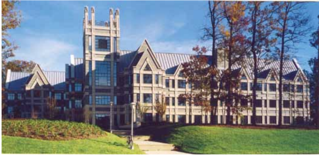
German limestone is anchored to precast panels on the Terry Sanford Institute of Public Policy at Duke University in Durham, N.C. (Architect Architectural Resources Cambridge Inc. )
