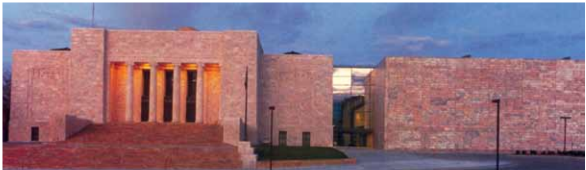
The new wing for the Joslyn Art Museum, Omaha, Neb. has 3 cm marble with 6 3 / 4 inch concrete backup. (Architects Sir Norman Foster and Partners ; Architect of Record: Henningson, Durham & Richardson, Inc. )
