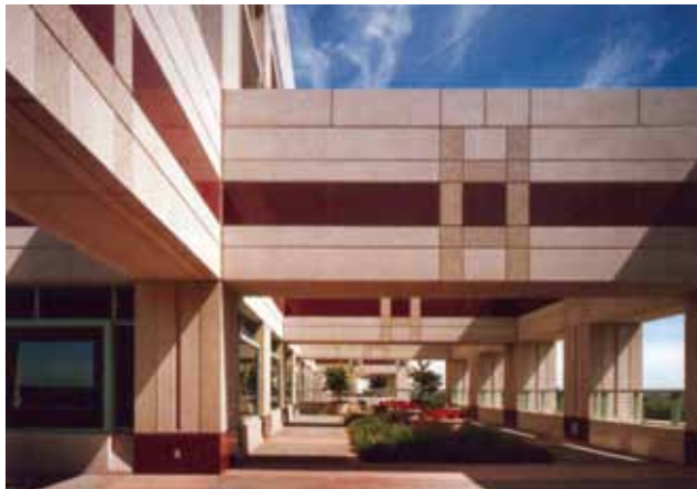
Polished granite feature strips on Shriners Hospital for Children, Sacramento, Calif. (Architect Odell Associates, Charlotte, N.C. and Associate Architect: HDR, Omaha, Neb. )
