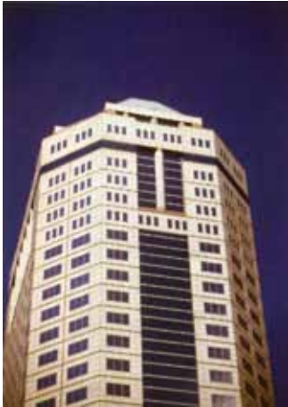
State Office Tower II, in Columbus, Ohio, has 3 cm of granite on 5- and 7-inch-thick precast concrete backup. (Architect Bohm-NBBJ)
