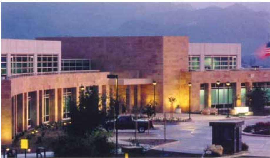
The Wellpoint Executive Center in Thousand Oaks, Calif., combines natural sandstone veneer-faced panels and precast to create a strong horizontal rhythm that blends into the hilltop.
