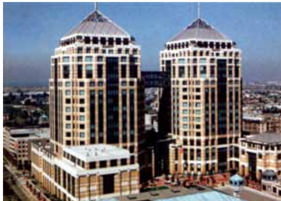
Two 18-story towers for GSA Federal Building, Oakland, Calif. are clad with 1- 3 / 4 inch beige and white-hued limestone. (Architect Kaplan McLaughlin Diaz)
