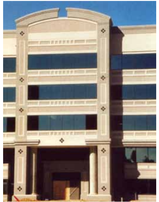
Black granite 8 inch square accents were used on the Munsell II office building in Alpharetta, Georgia. (Architect Harris-Fritz Architects )
