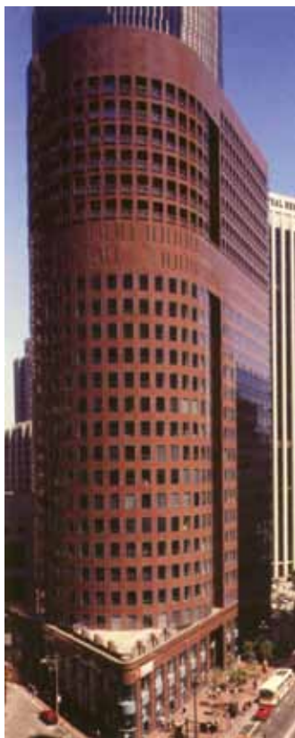
388 Market Street building in San Francisco, Calif. is clad with 3 cm granite anchored to precast concrete. (Architect Skidmore Owings & Merrill )
