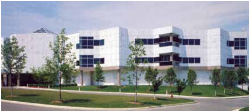
Hospital Corporation of America's Data Center, Nashville, Tenn. has 1 inch thick marble on a 5 inch precast concrete backup. (Architect Gresham, Smith and Partners )
