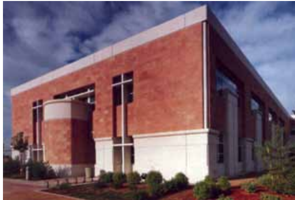
Precast concrete panels are integrally cast with Arizona Red sandstone on the Roseville Telephone Company in Roseville, Calif. (Architect Williams & Paddon Architects & Planners, Inc. )
