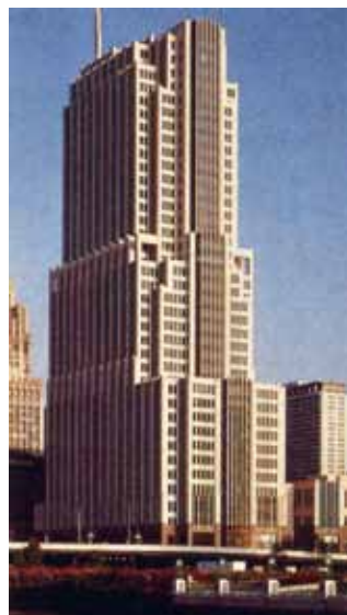
NBC Tower at Cityfront Center, Chicago, Ill. has 2 or 2 3 / 4 inch thick limestone on 5 inch thick precast concrete backing. (Architect Skidmore, Owings & Merrill )
