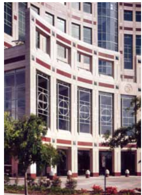
Panels on the Shriners Hospital for Crippled Children, Sacramento, Calif. are 6 inch thick and have a horizontal band of 3 cm granite attached with one anchor per 2 sq. ft. (Architects Odell Associates ; and Associate Architect: HDR )
