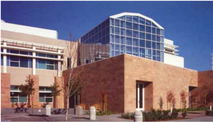
Arizona red sandstone, 3 cm to 1 3 / 4 inch thick, was anchored to 4 inch thick concrete panels for the Sacramento Municipal Utility District's Customer Service Center, Sacramento, Calif. (Architect Williams + Paddon Architects & Palnners, Inc. )
