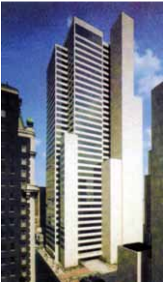
Southwestern Bell, Dallas, Texas has 3 cm travertine anchored to 7055 precast concrete units. (Architect JPL Architects)
