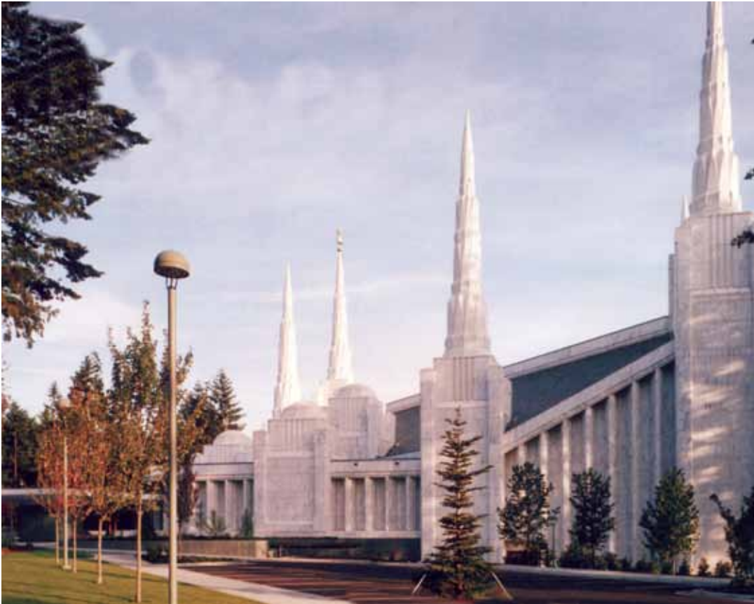
The base structure of the Portland Oregon Temple for the Church of Jesus Christ of Latter Day Saints, Lake Oswego, Oregon consists of 3 cm marble facing backed with 4 inches of precast concrete. (Architects Lee, Ruff, Stark Architects; and Leland Gray Architects )
