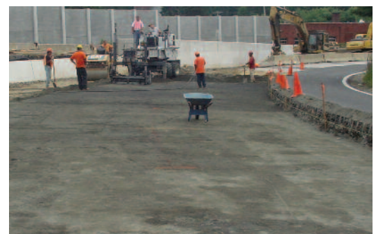
Warped slabs (above) are required for three-dimensional highway surfaces
