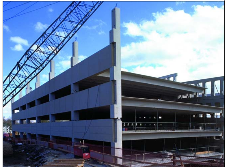
Double Tees provide uninterrupted long- spans for this water treatment facility.
