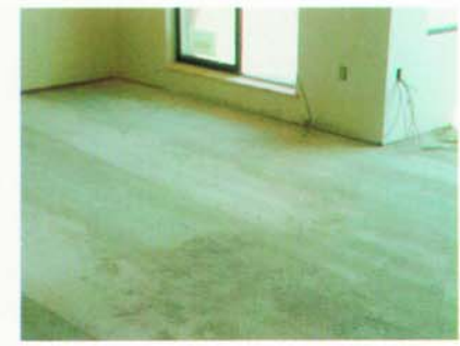
Top surface prepared to receive flooring materials.
