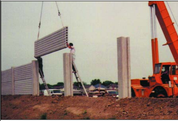
Sound barrier walls.
