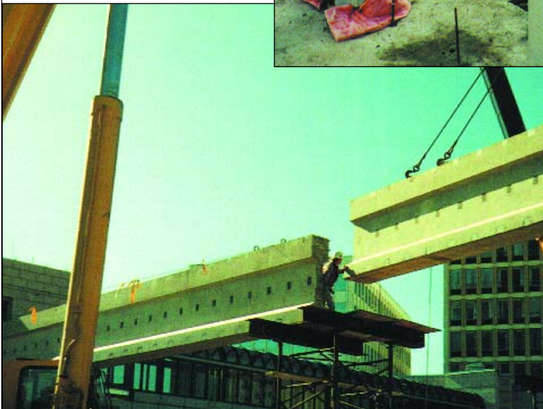
Post tensioned transfer beam.
