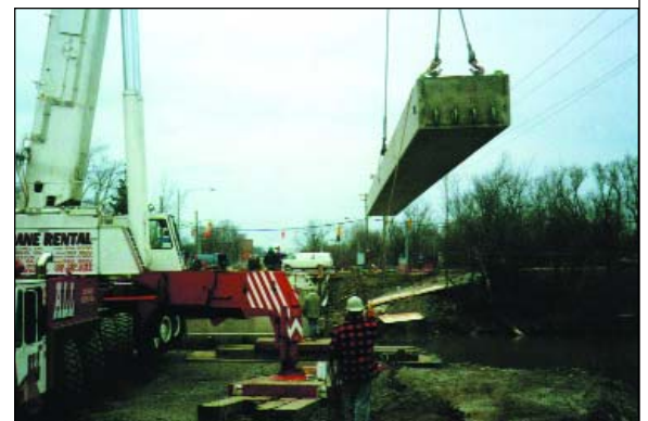
Standard girder sections minimize engineering and manufacturing time, resulting in quick product availability.
