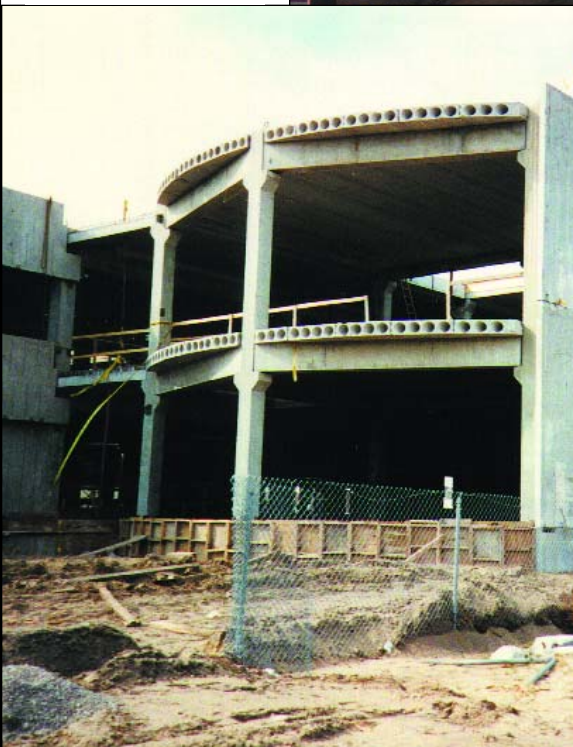
Versatile hollow core units can be designed to suit many applications.
