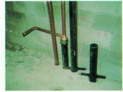
Pipe installation and sealing by mechanical trade follows core drilling.
