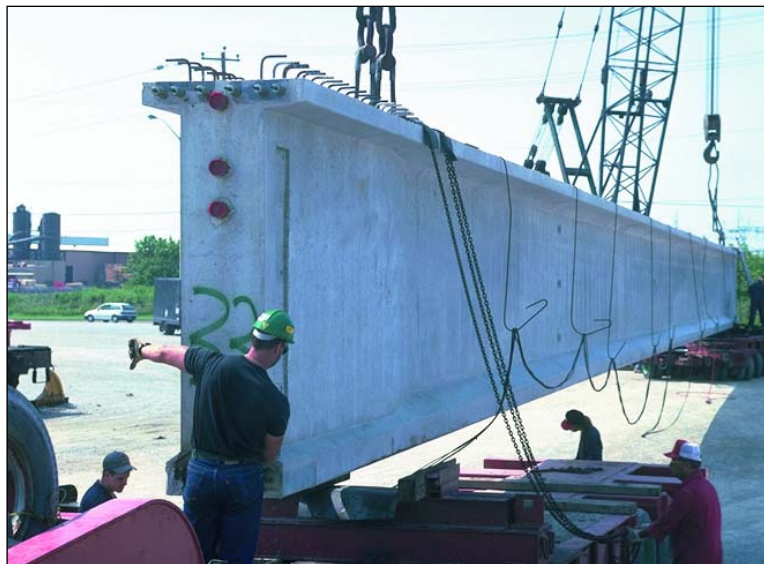
Standard girder sections minimize engineering and manufacturing time, resulting in quick product availability.
