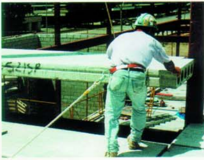
Individually identified units being installed.
