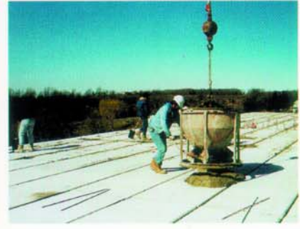
Grouting of shear key for load transference.
