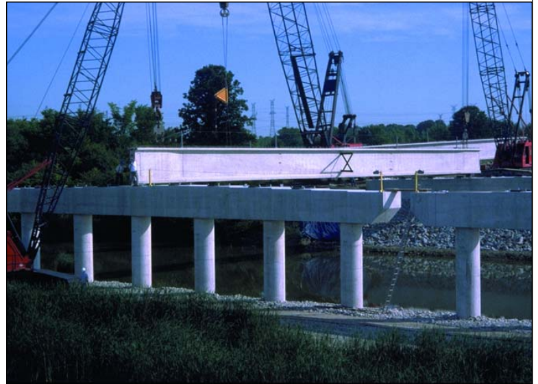
Plant cast girders are quickly placed during off-peak times, minimizing traffic interruption.
