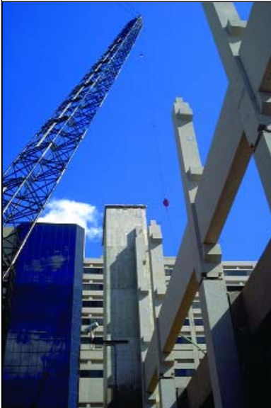
Multi-level beam and column framing
