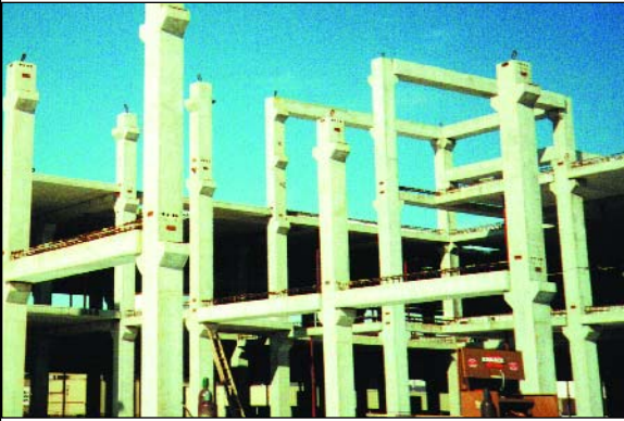
Framing is quickly assembled immediately after site work.
