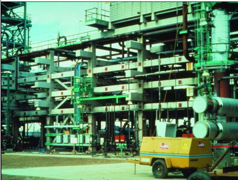
Precast pipe racks.
