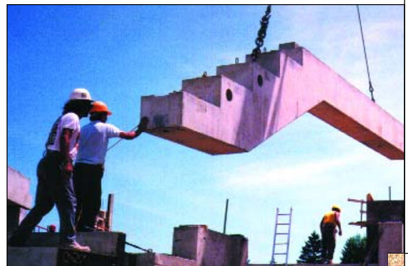
Placement of a raker beam.
