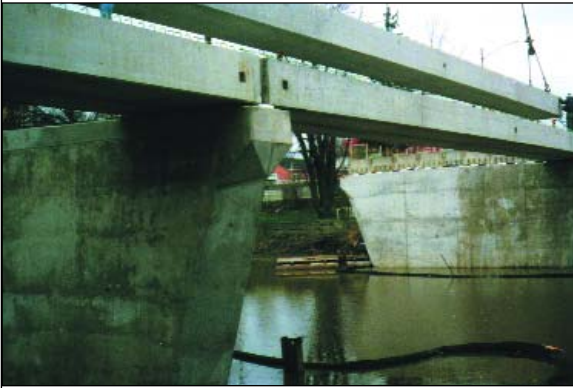
Plant cast girders are quickly placed during off-peak times, minimizing traffic interruption.
