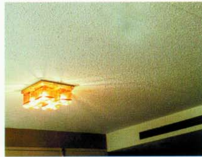
Attractive stippled exposed ceiling.
