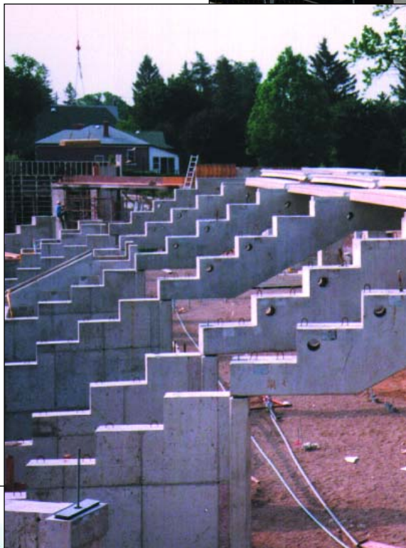
Precast concrete raker beams are ready to receive bleacher seating.
